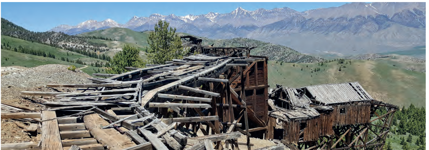
800 level historical ore load-out
