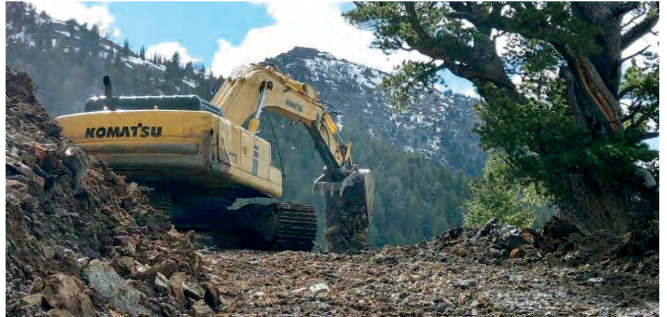
Drill road construction
